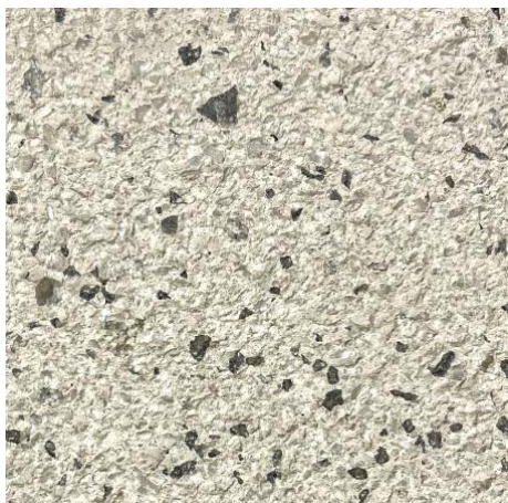
56 Bush-hammered concrete ASSEN
